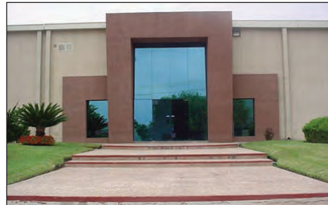
Monterrey, Mexico Manufacturing and Distribution
